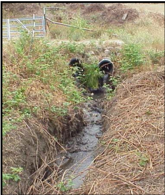
Wrights Creek - Proposed site for fish passage barrier removal
