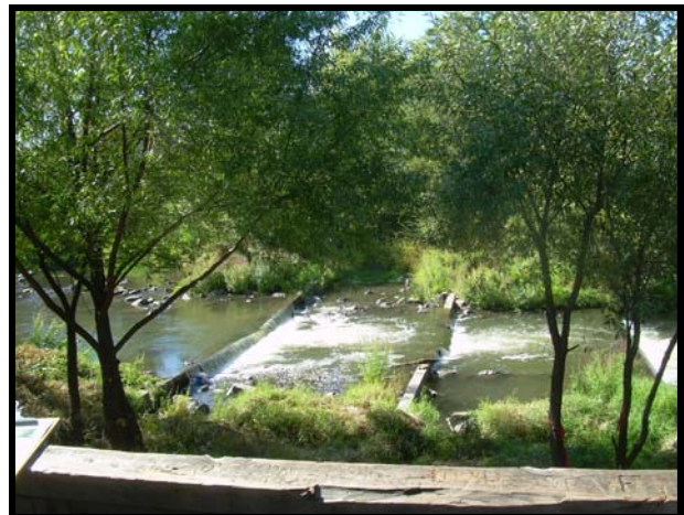
After maintenance and vegetation removal
