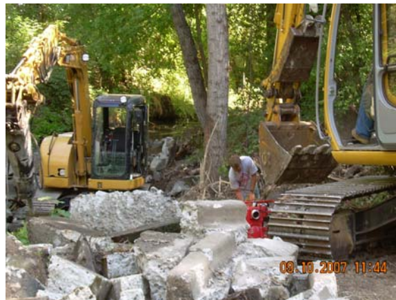
Dam structure removed from Lazy Creek bed.
